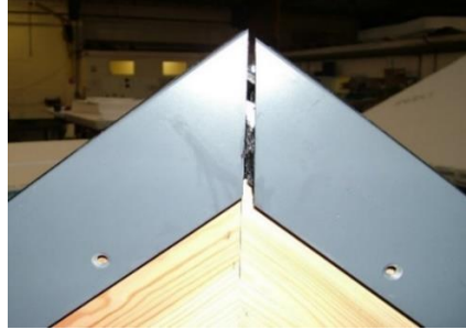
Figure 12 – The second section is lowered to meet the first section at the apex
